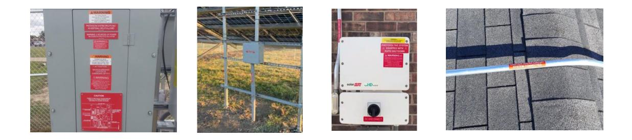
Labeling: Photos showing clear and accurate labeling is present as necessary on inverters, disconnects, conduit, Main Service Panel, and other electronics. As part of the review, additional labeling photos may be requested as part of the system review.
