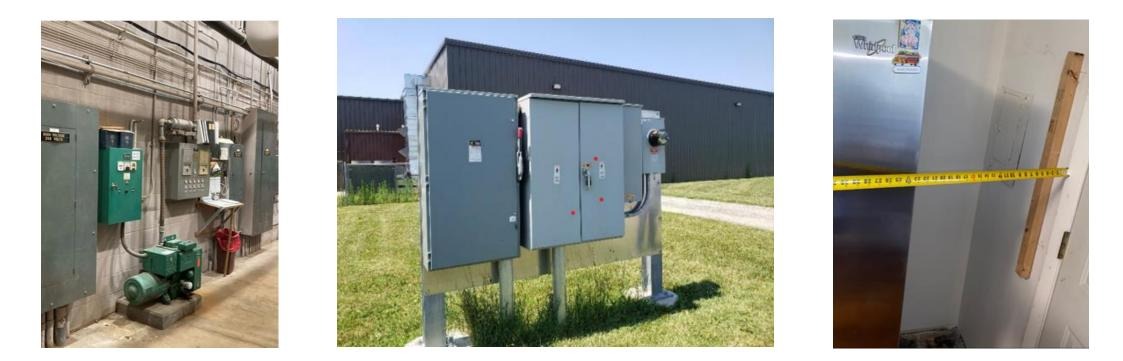
Area Clear of Obstruction: Photos showing the condition of the area surrounding the electrical panels. It is important to show multiple photos. Additional work to ensure a clear work area should be noted as part of the site's suitability.
