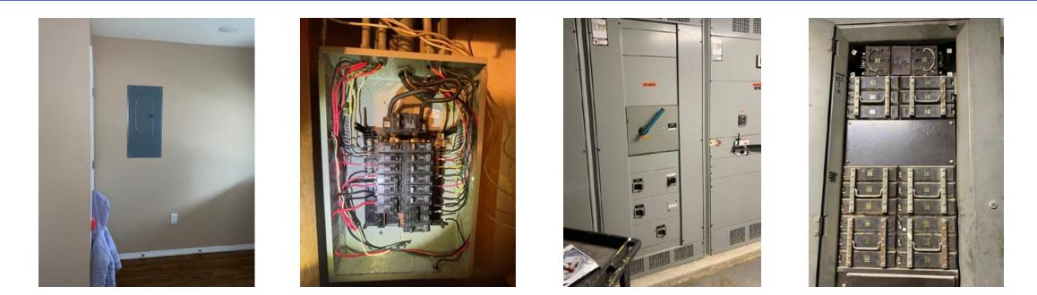
Photos showing the condition of the electrical panel at a Residential Solar (Small) location and Non-Profit Facility. It is important to show multiple photos. One with the Main Service Panel cover on and visible and another with the cover removed exposing the service and branch wiring. See the Electrical Assessment section of the Site Suitability Guidelines.
