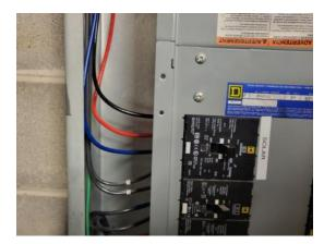
Load Side connection: photo showing the wiring connection of the PV system through a UL listed and properly rated back-fed breaker in the main service panel. Supply Side: a photo showing a properly rated, UL listed tap was performed for the connection to the switch board or main service panel.
